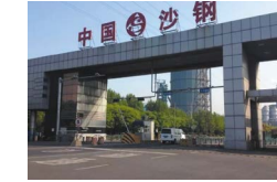
Jiangsu Shagang Iron and Steel, Jiangsu, КНР стр.52
